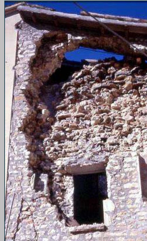
Separation of leaves in a repaired stone masonry
