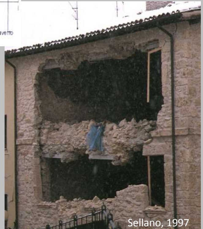
Expulsion of the façade: the tie-beam is supported only by the internal leaf of a multi-leaves masonry: load eccentricity and reduction of the resisting area
